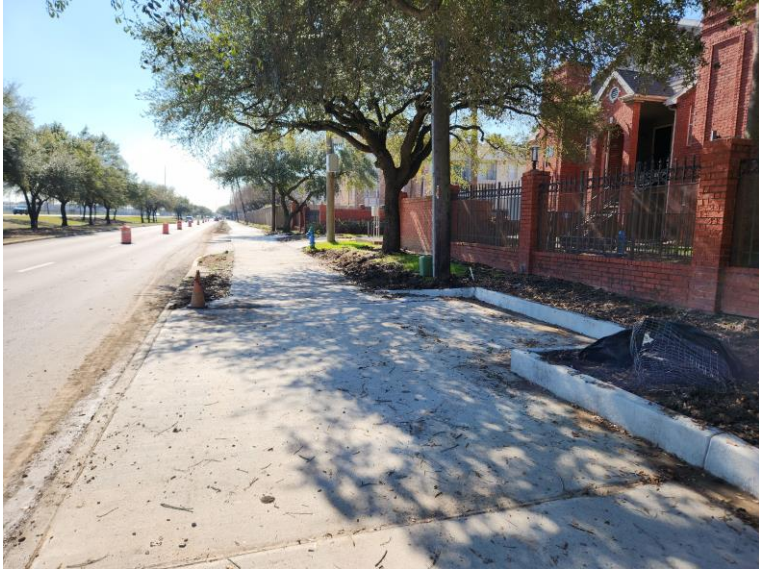
Existing Pad Conditions
